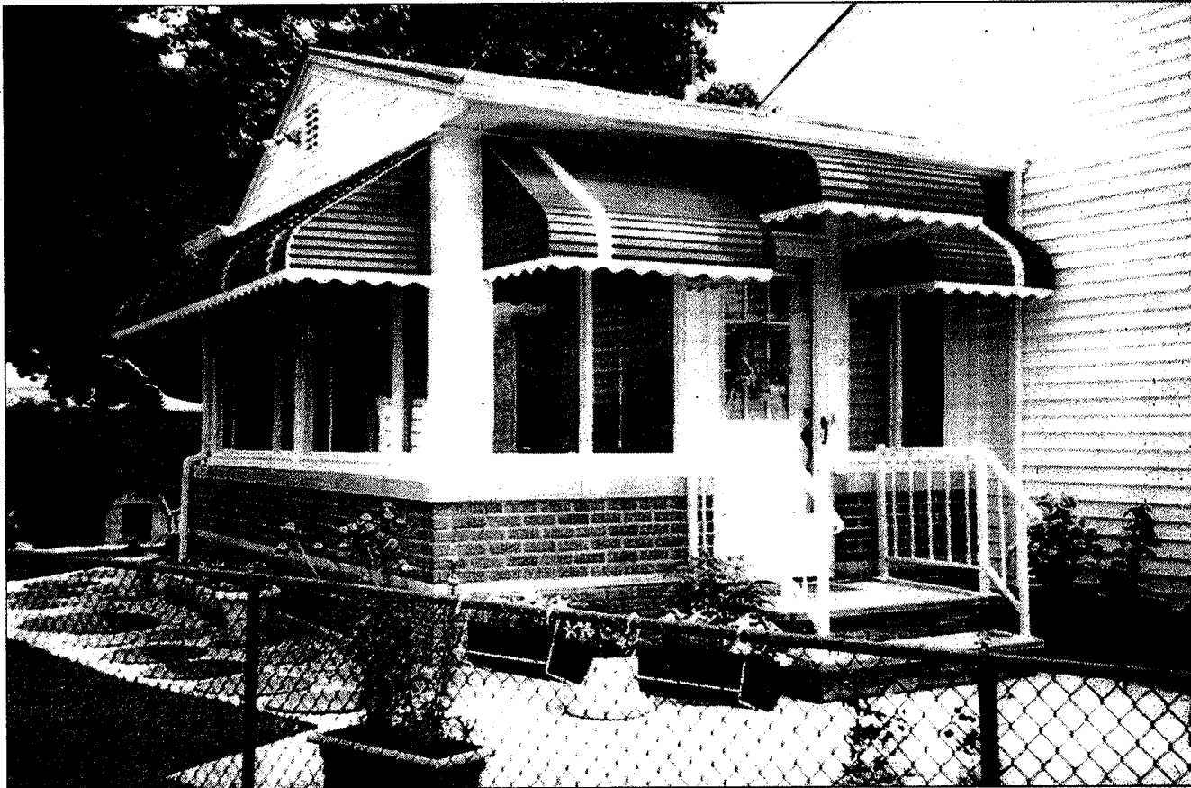
These awnings were custom-built to fit the various sizes and styles of windows. Proper sizing of awnings is important both for blocking the summer sun and for allowing the winter sun to shine through the windows for passive solar heating.
