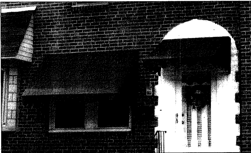
Fabric awnings with sides can block the sun throughout the day. Some that are adjustable can also be raised to almost completely expose the window glass.
